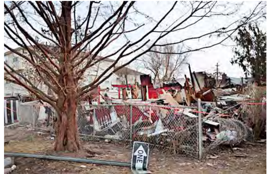
Damage from Hurricane Sandy
